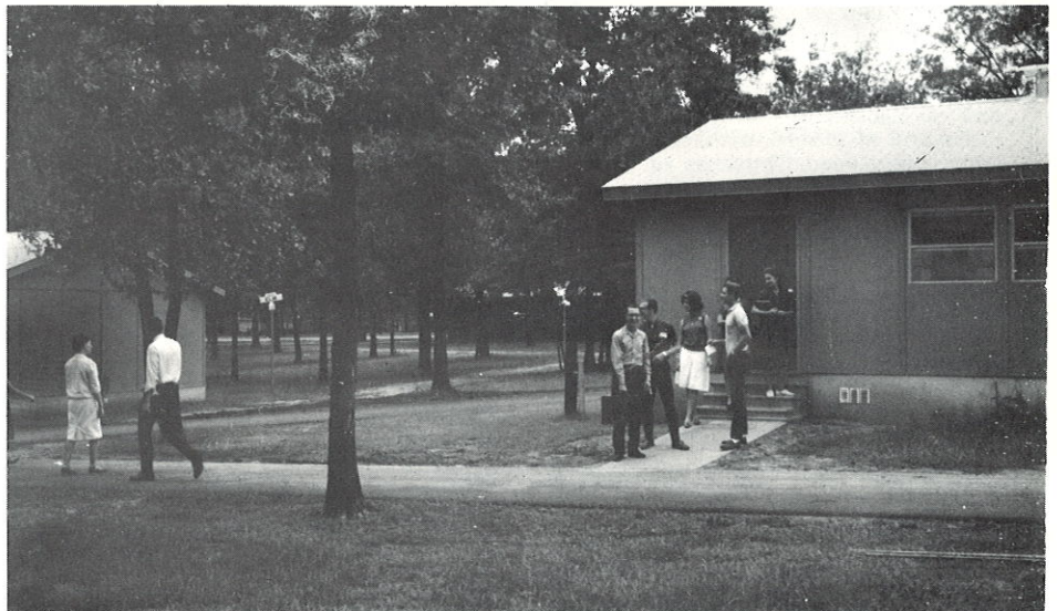
Studies Begin in Temporary Classroom Buildings
