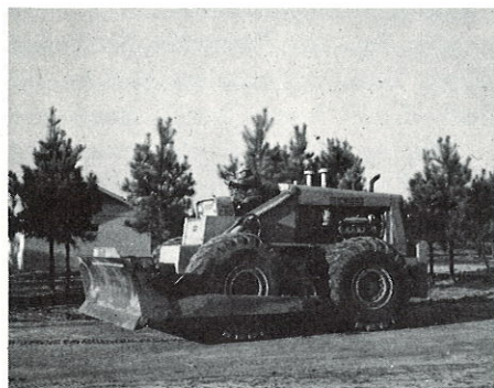
Dozer Ready for Action
